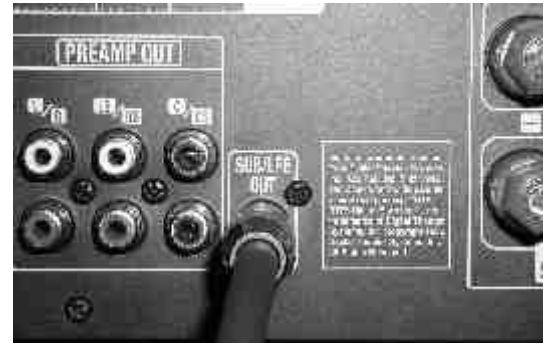
RCA connection from Processor to a Kompressor using a "Y" connector.
